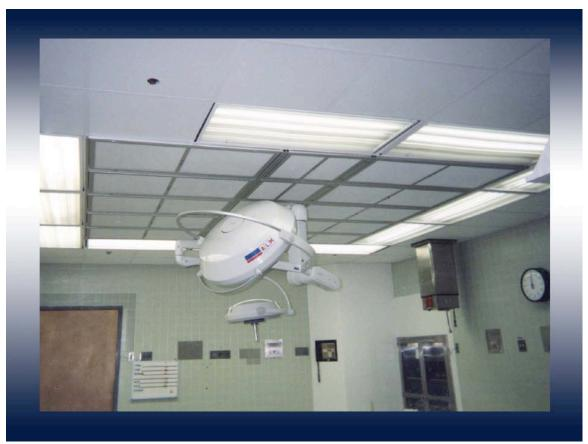
he key to achieving contamination control, whether in the hospital operating room or the semiconductor assembly area, is the air filtration system, which is ultimately dependent on the reliable performance of HEPA (and in some cases ULPA) filters. This includes cleanrooms and mini clean filtration "environments" such as biosafety cabinets, clean benches and fume hoods.
